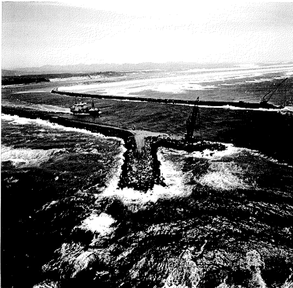
Figure 28. Construction of spur jetties at the entrance to the Siuslaw River, Oregon, 1985.
