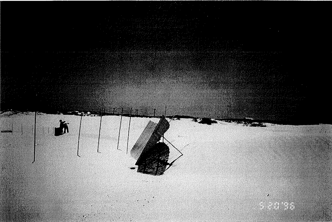
Figure F11. Sand fencing at Packery Channel. Upper photo: sand dune development adjacent to a sand fence a few days after installation. Lower photo: severe scour at the base of a fence.
